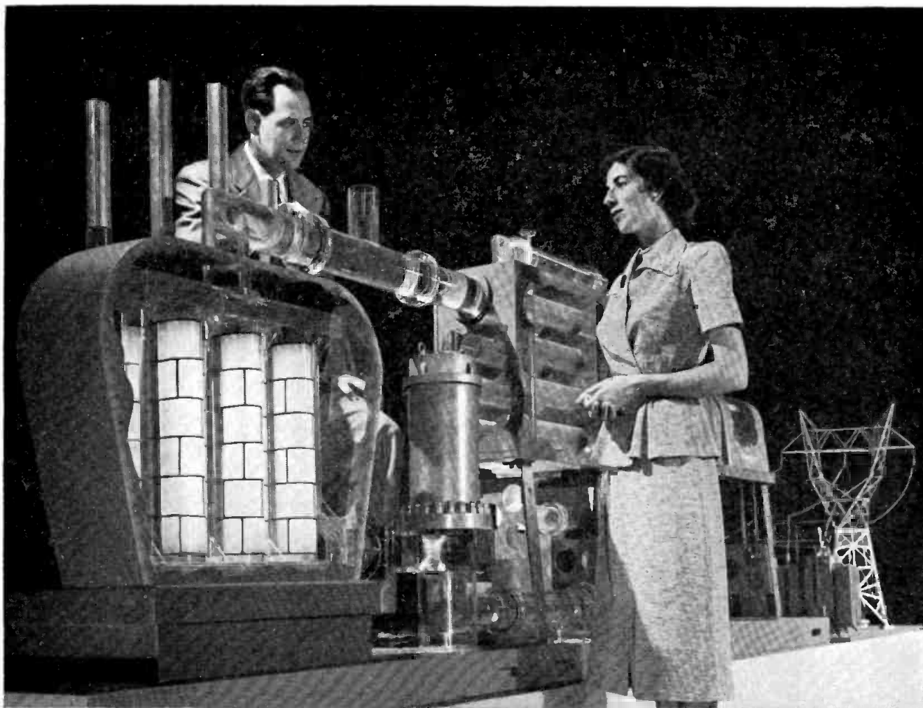
Richard Noble and his wife inspect a small model, about 1/30 actual size, of the nuclear power plant he is helping to design. This plant, except for its heat-producing unit (foreground), will look much like any other power plant. It is to serve as a "laboratory" from which much will be learned about using the atom as a fuel to help fill future needs for more and more electricity.
